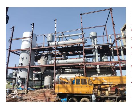
500 TPD soybean preparatory and continuous solvent extraction plant in West Africa, designed for high-quality soya flakes and collets production
