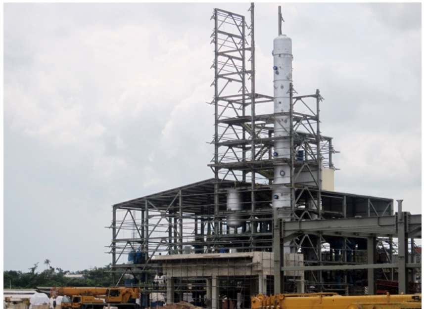
100 TPD Continuous Physical Refinery for crude palm and palm kernel oil in Nigeria
